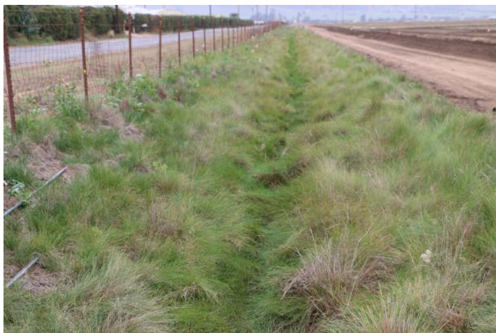
Figure 7. Permanent ditch planted with red fescue can infiltrate run-off and protect the sides of the ditch from eroding during large storm events. This ditch is located at the USDA-ARS along Spence Road in Salinas.
